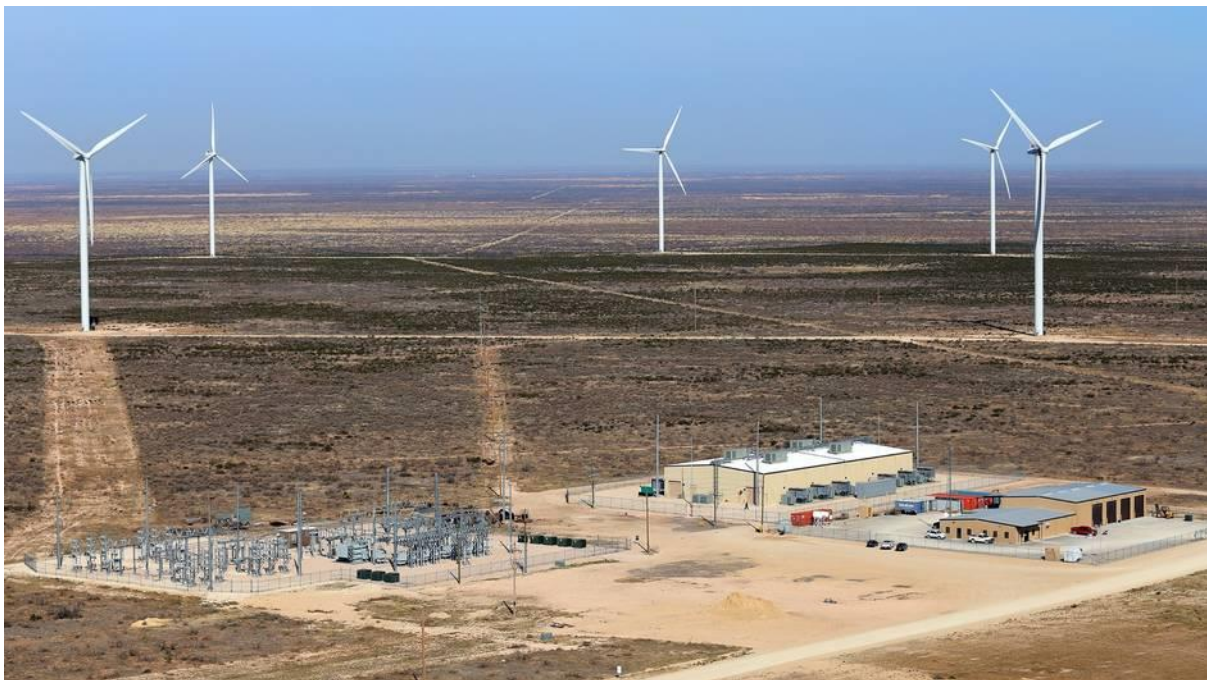
Figure 1-13: Duke Notrees Storage Facility in Texas
