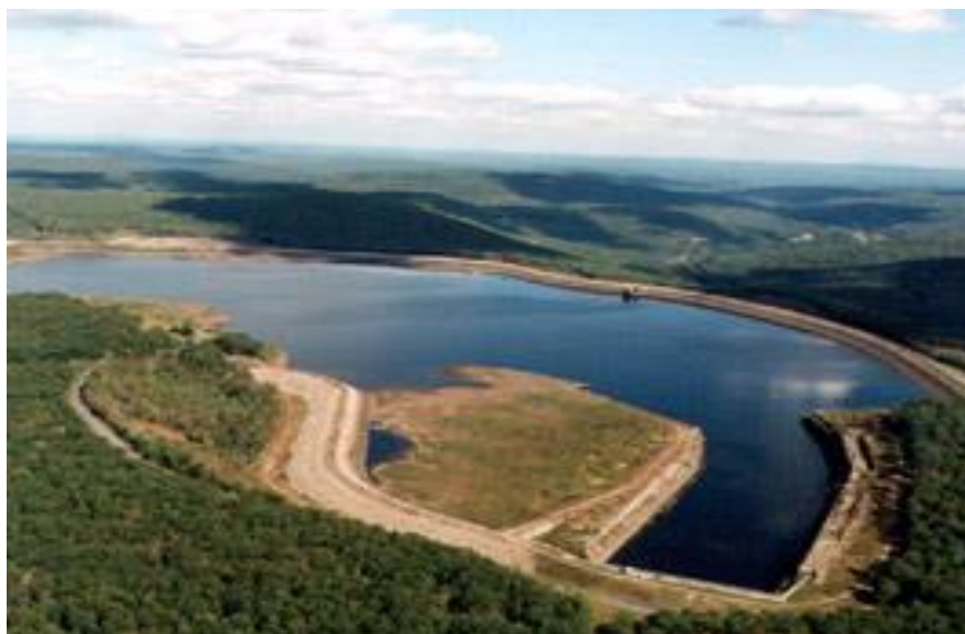
Figure 1-2: Northfield Mountain Pumped Storage Project in Massachusetts
